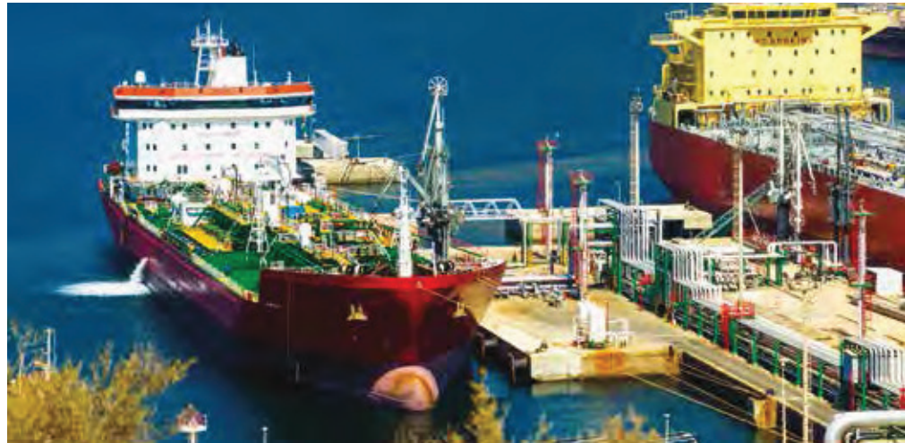
The main challenge for a BWMS with side-stream dosing is the location of the treatment system and the resulting piping arrangement for motive water
